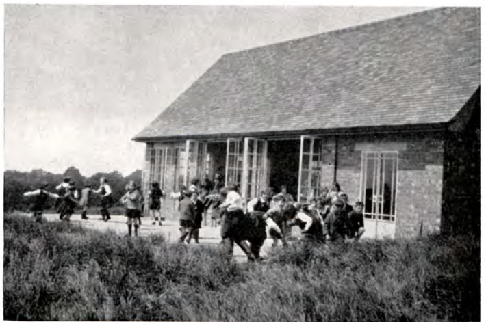
A CLASSROOM ON THE WYTHAM UPLANDS Note the two large windows that fold and slide right back. This type of classroom, 42ft. by 20ft., cost £525
